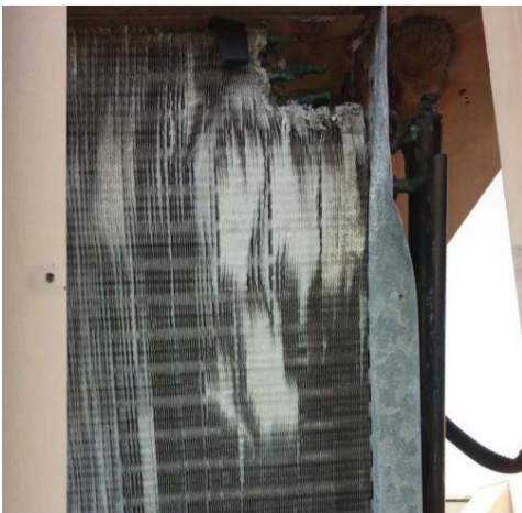
Figure 3: Condenser coil before Ener.co ® treatment
